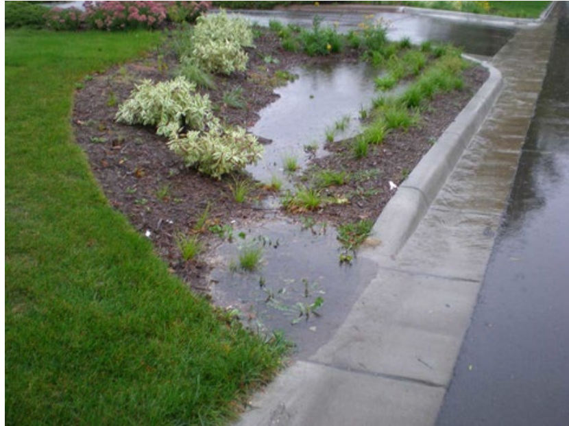
Figure 4 shows a rain garden. Rain gardens are one type of LID that is used to help stormwater management systems by absorbing excess water and filtrating run-off. https://extension.umn.edu/landscape-design/rain-gardens
