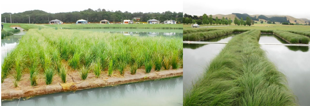
Figure 3) These are both images of constructed floating wetland systems (Martin Ecosystems; Atlan Stormwater).
