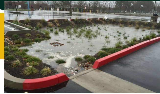
› A bioretention planter on the Sacramento State campus.
