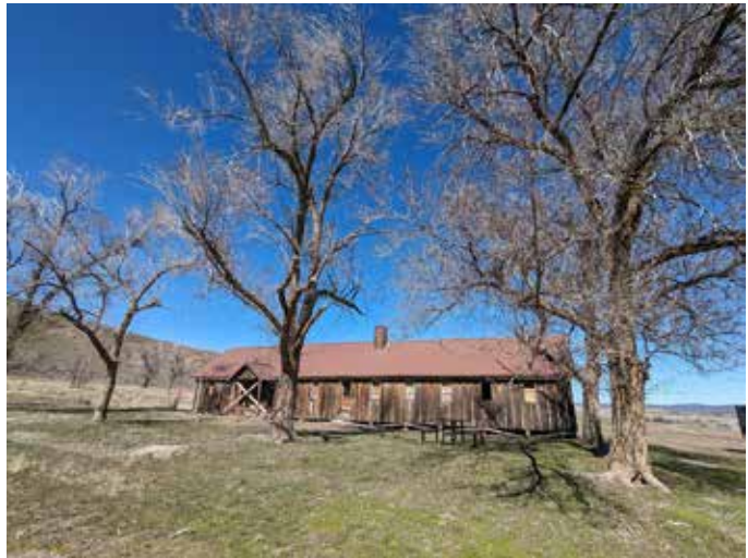
The mess hall and kitchen.
